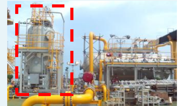
Two-Stage CFU tied directly into separator
