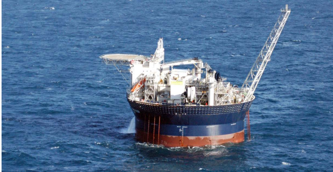
Figure 16-2 Western Isles FPSO Sevan 300 Unit
