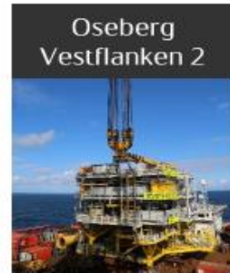
Ongoing In operation Unmanned Wellhead Platform (UWP™)
