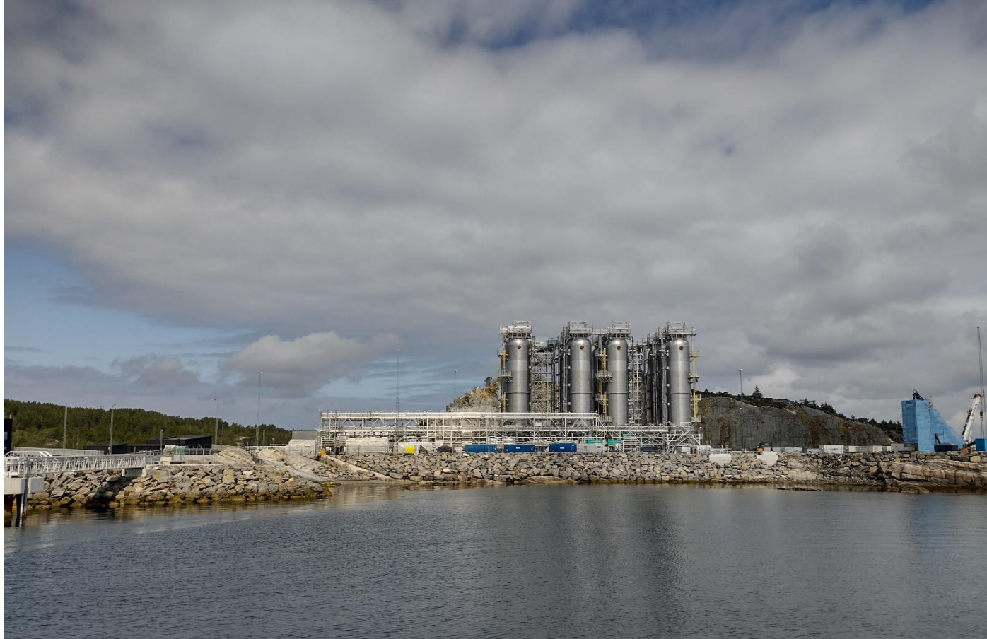
Northern Lights onshore facilities at Øygarden, Norway
