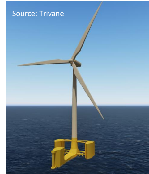
Trivane hybrid steel/concrete barge
